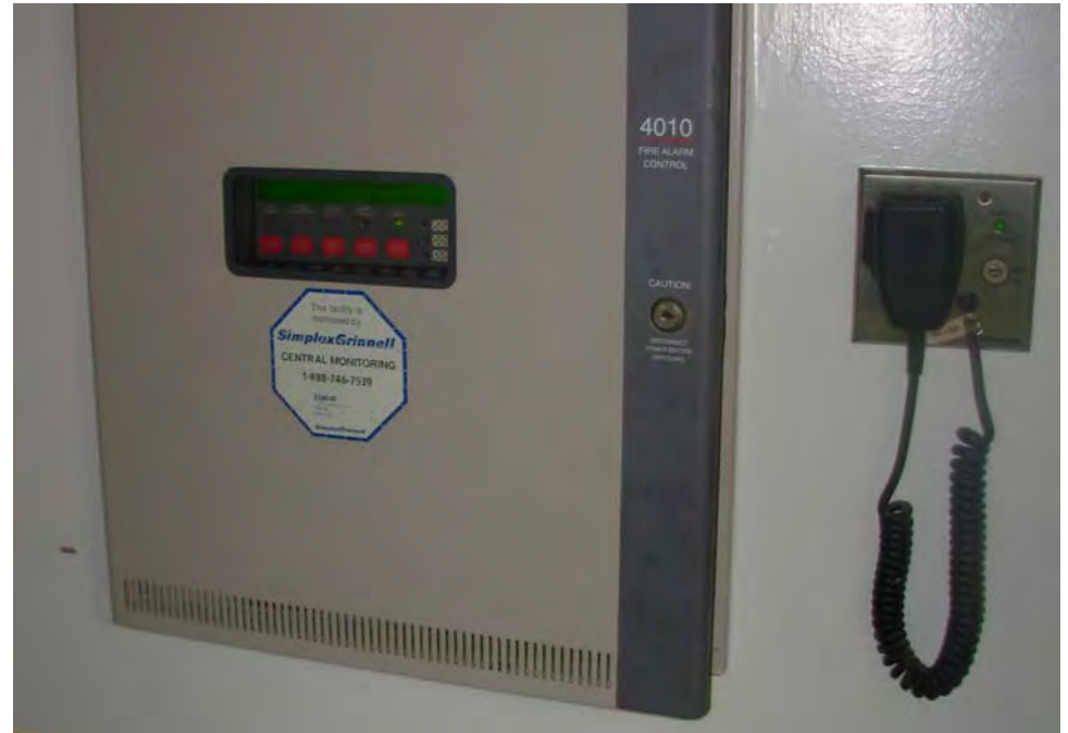
32. Fire detection - monitoring serving daycare facility
