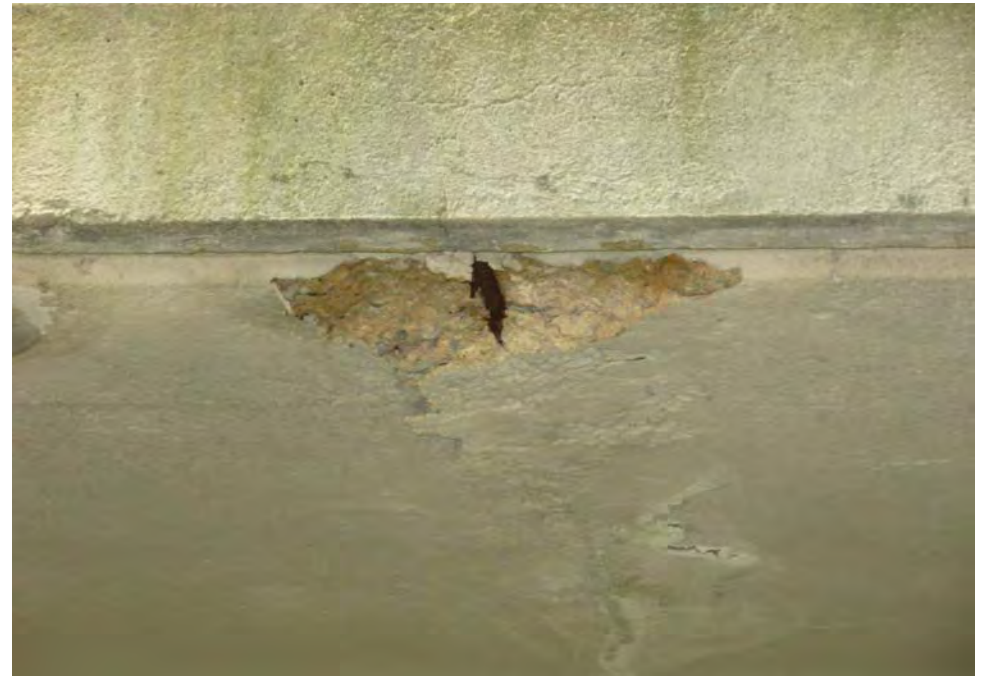
12. Spot rebar exposure at balconies
