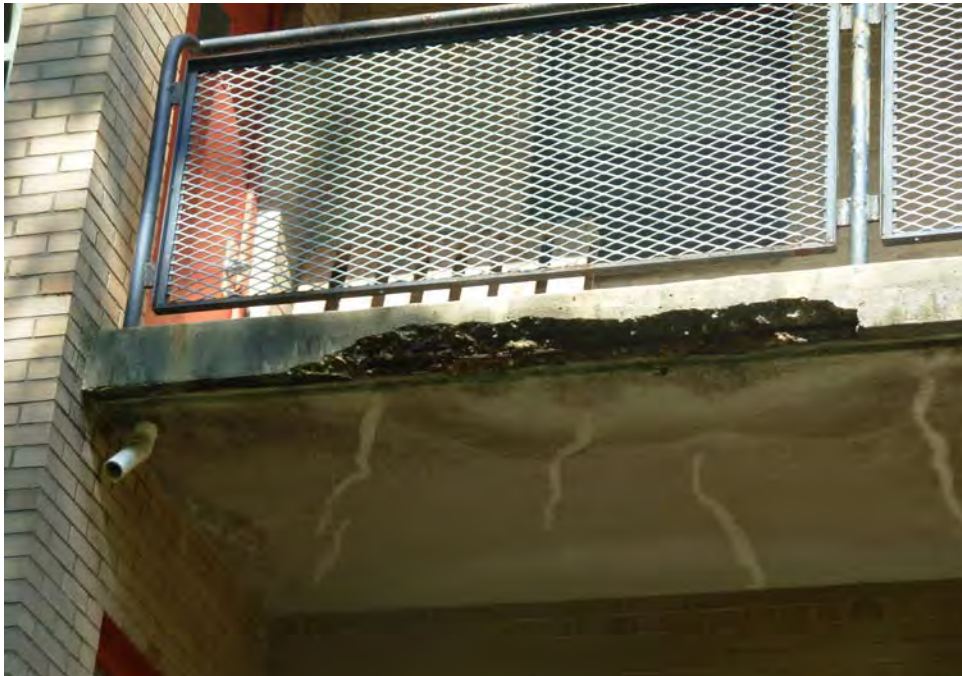
11. Spot spalling of concrete balconies
