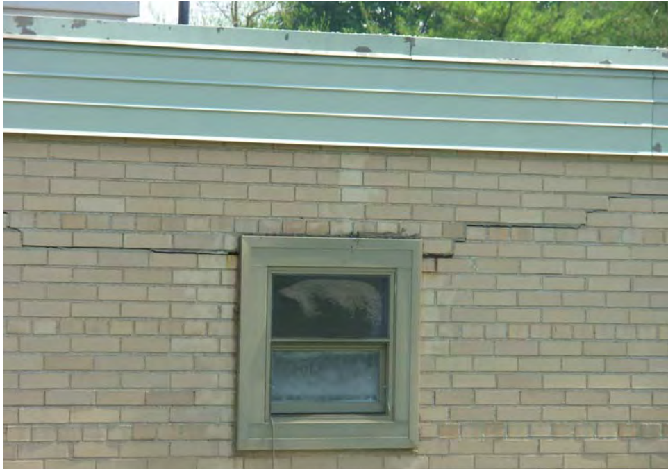
13. Spot masonry cracking and mortar deterioration
