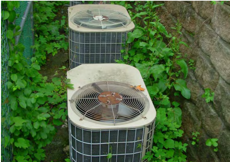
31. AC condensers serving First Steps HVAC systems
