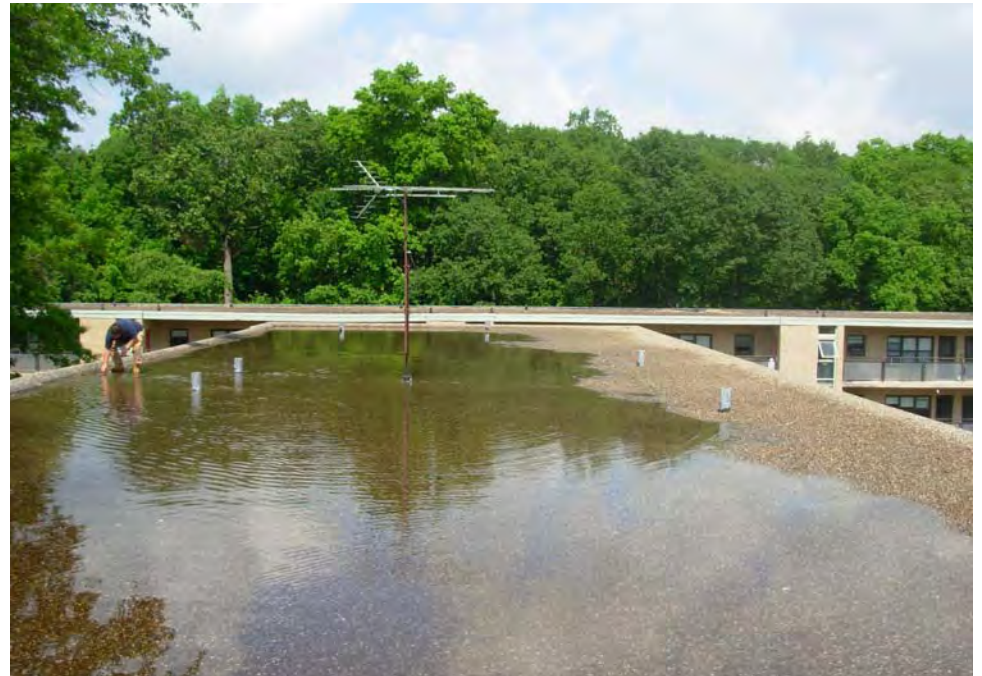
16. Ponding at one roof surface, due to clogged drains and poor pitch
