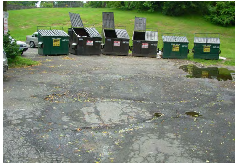
4. Paving at dumpsters, poor conditions
