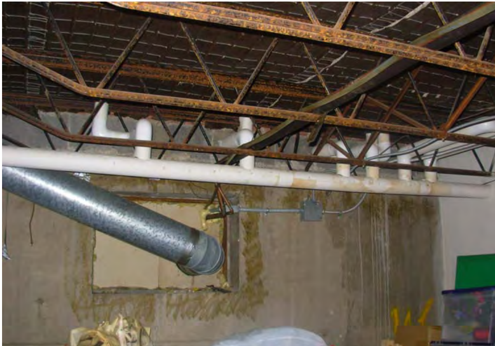
27. Basement-crawl space structure and distribution piping
