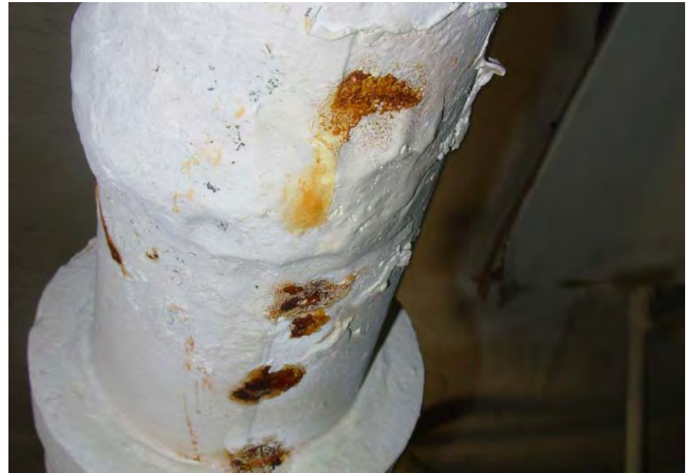
28. Spot leaks of heating and DHW service line piping
