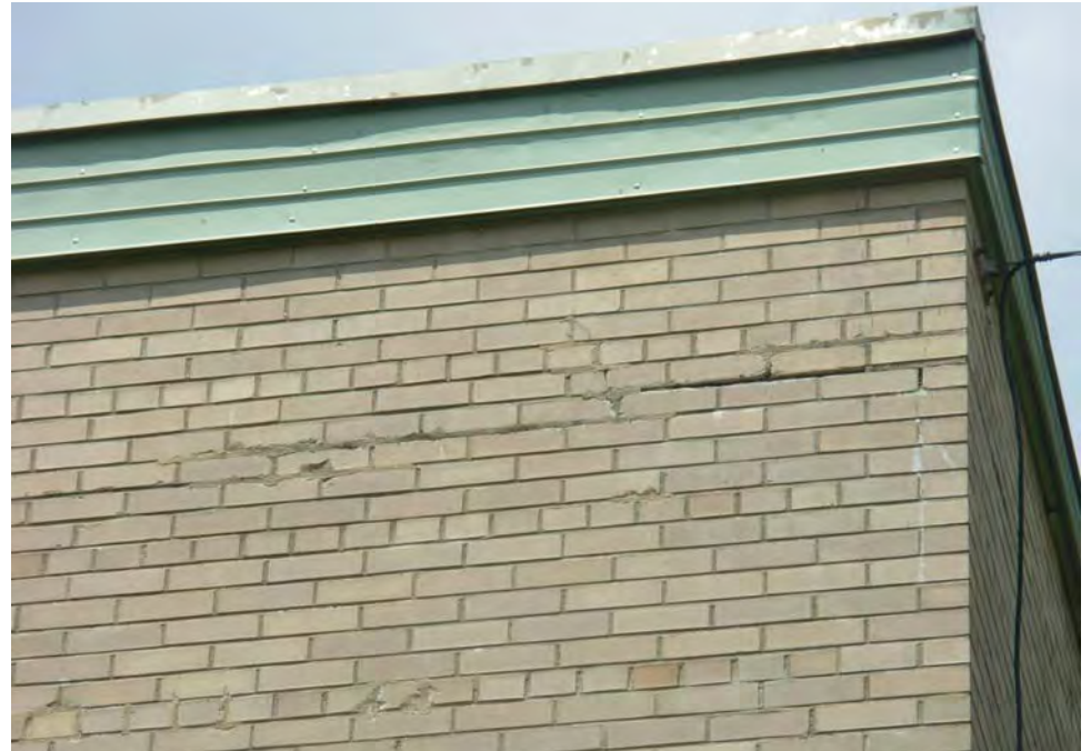
14. Spot mortar deterioration, patch repairs done
