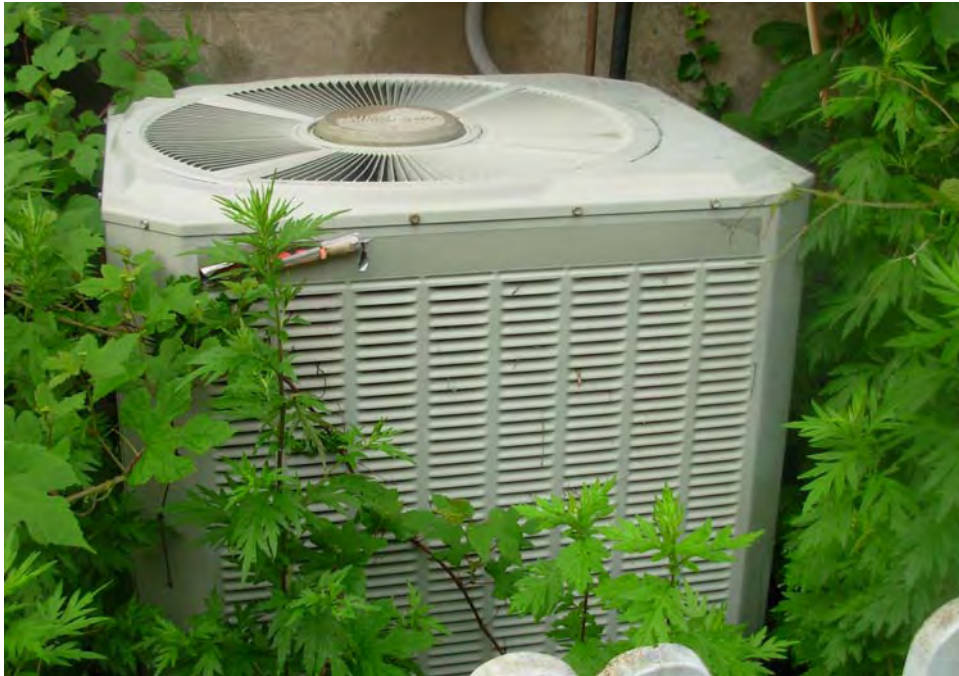
29. AC condenser serving Kids Corner daycare - to replace
