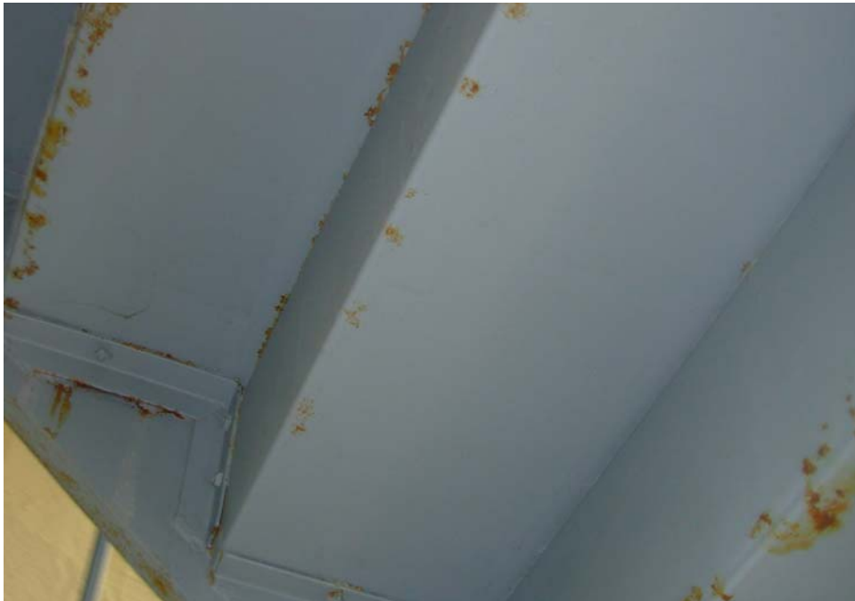
23. Some rusting of stair structures
