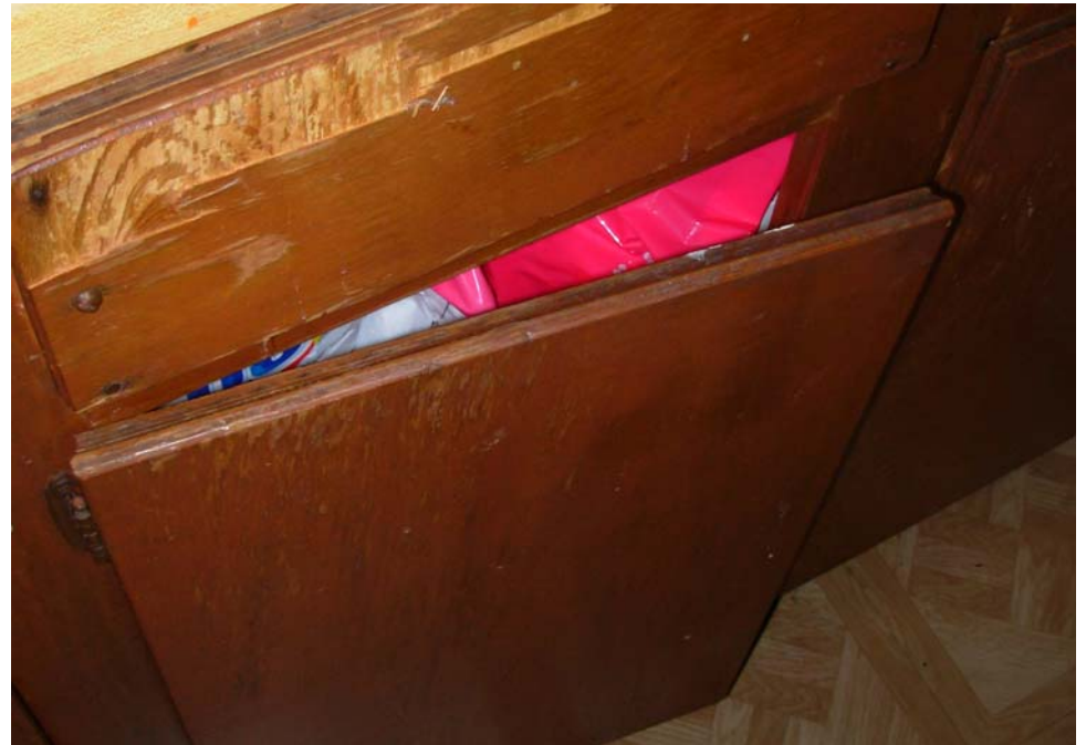
36. Spot damage and deterioration of kitchen cabinetry
