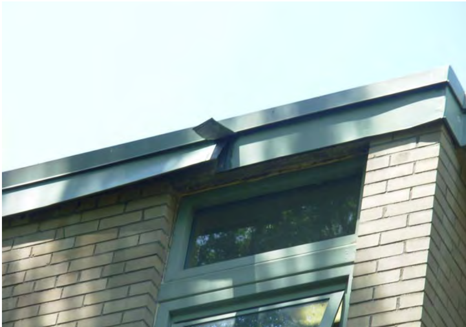
15. Some roofing fascia flashing damage
